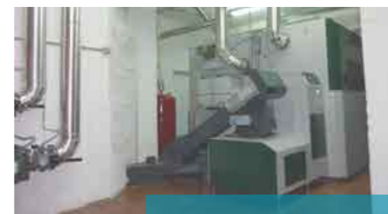
Biomass boilers and adapted to work with pellets, wood chips, olive stones, cuttings, etc.
